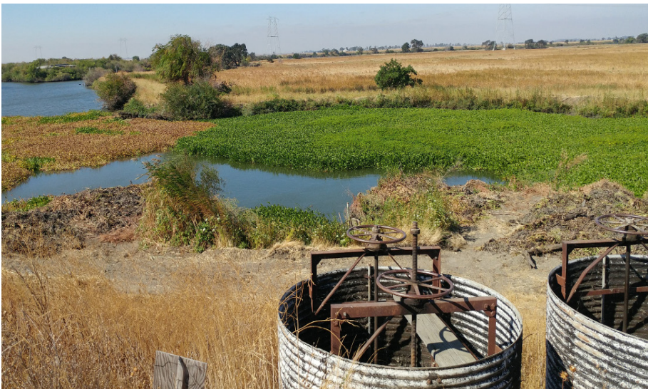
View 3. View of the Vogel Property looking south from the Cache/Hass Slough Levee where Cache Slough connects via screw gates to Lookout Slough.
