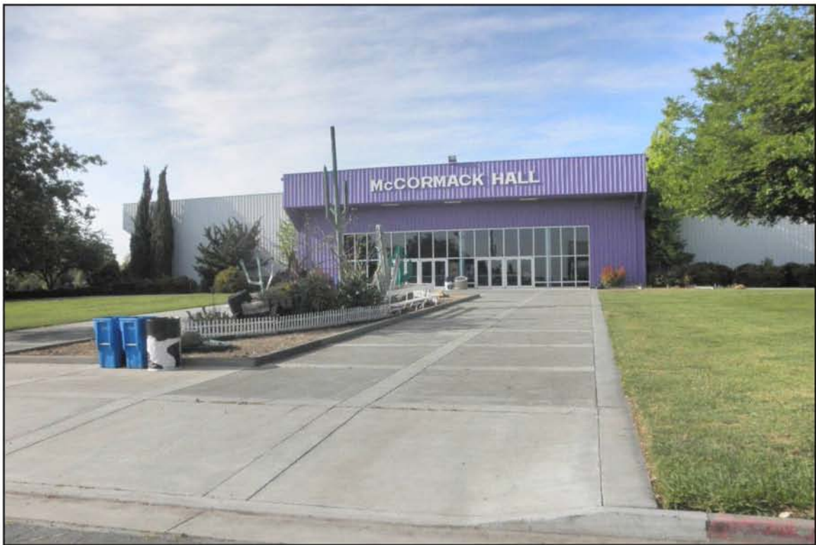
Photograph 13: McCormick Hall; facing north.
