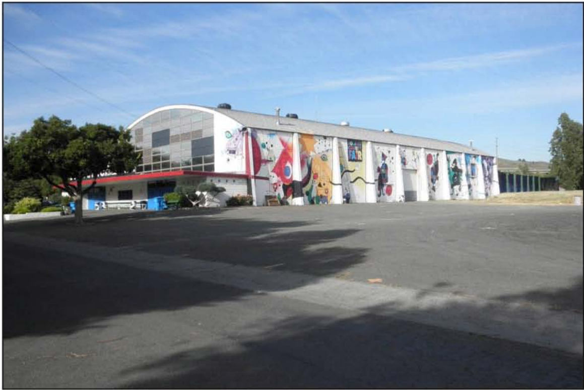
Photograph 11: Exposition Hall; facing northeast.
