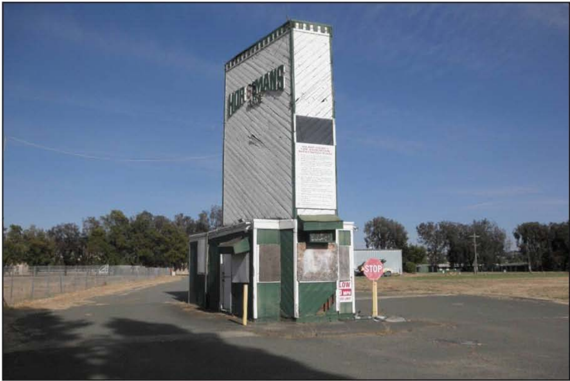
Photograph 7: Horseman's Cafe sign marking entrance to racetrack; facing east.
