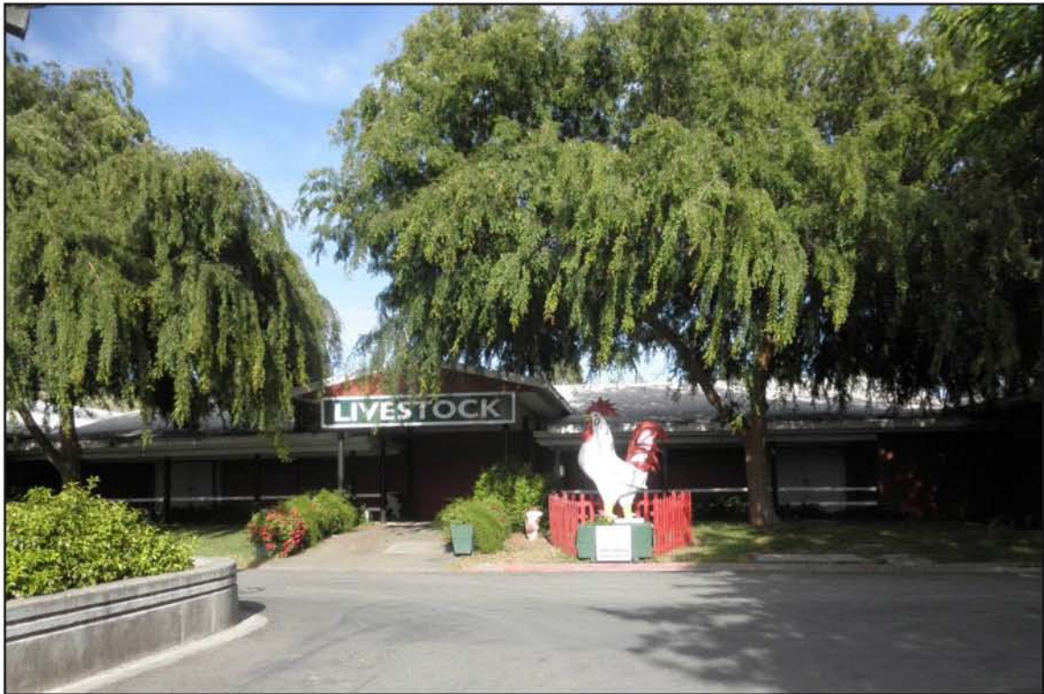
Photograph 12: Livestock Building; facing east.
