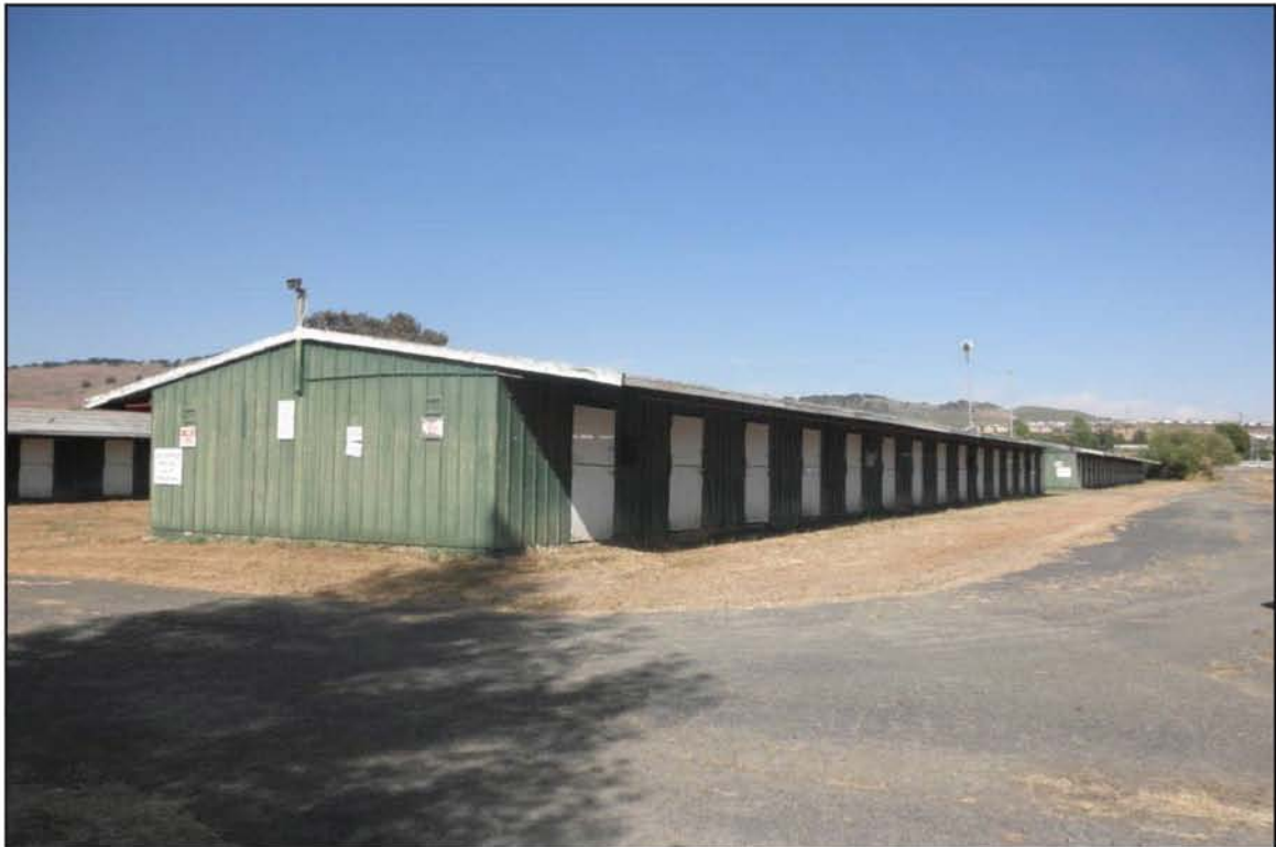
Photograph 2: Detail of stables; facing northeast.
