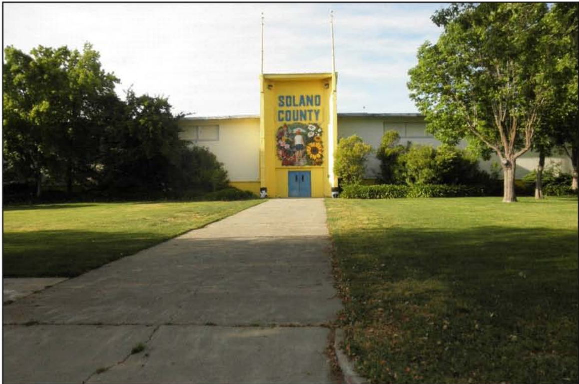
Photograph 14: Solano County building; facing north.
