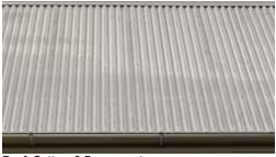
Roof, Gutters & Downspouts Corrugated metal roof half-round metal gutters, gutter straps every other rail; mt-factory-applied Charcoal Gray Color
