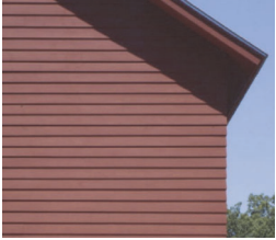
Siding, Fencing & Gates STK Cedar, 1x vertical T&G and 1x horizontal ship lap Painted barnyard red; Fences/gates not to exceed 6' tall
